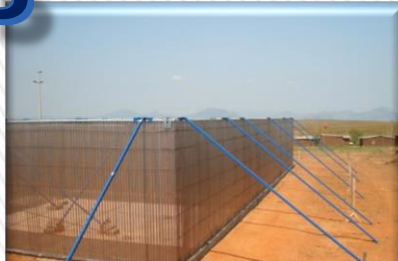
Erection of wall panels
