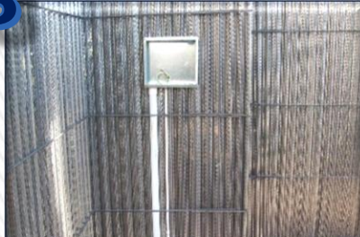
Fitment of In-wall electrical services
