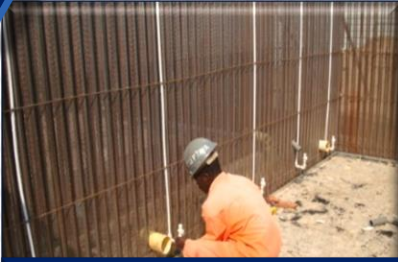
Fitment of In-wall plumbing services
