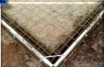
Preparation of Raft Foundation
