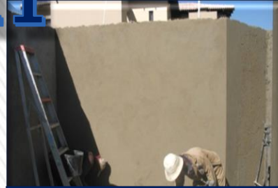
Plaster finish to mortared walls
