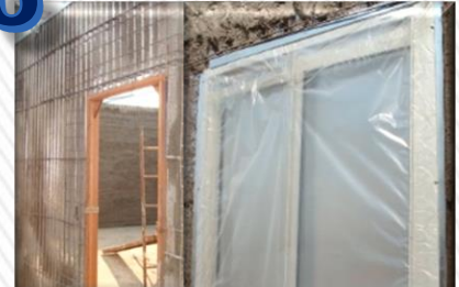
Fitment of door and window frames
