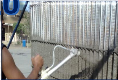
Mechanically applying mortar to walls
