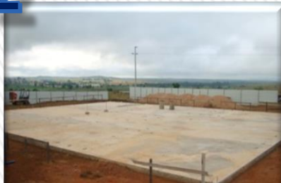
Casting of Raft Foundation
