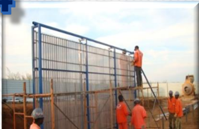
Assembling Wall Panels
